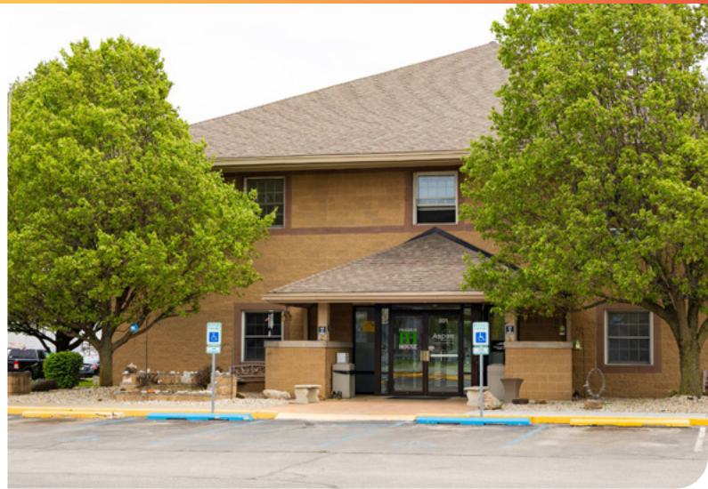
Aspire's Progress House Recovery Center in Indianapolis
